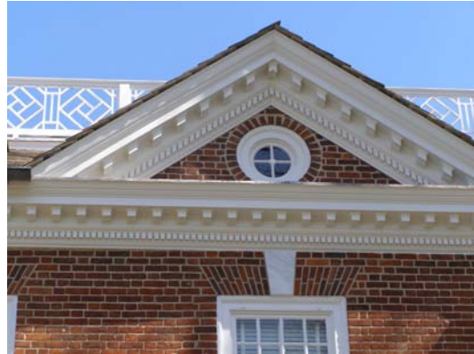
Cornice after restoration.
