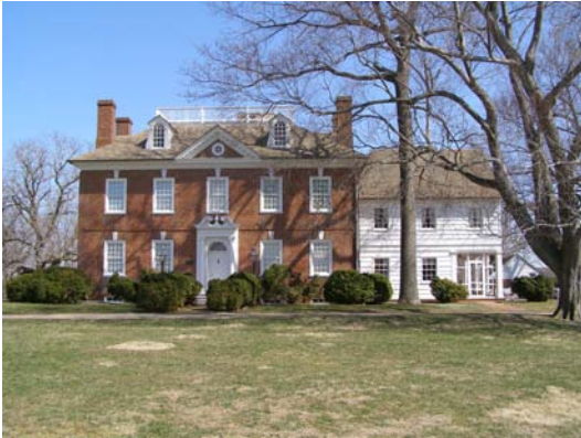
Manor House after restoration.
