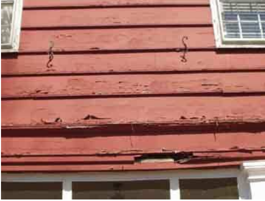
Clapboard addition before restoration.
